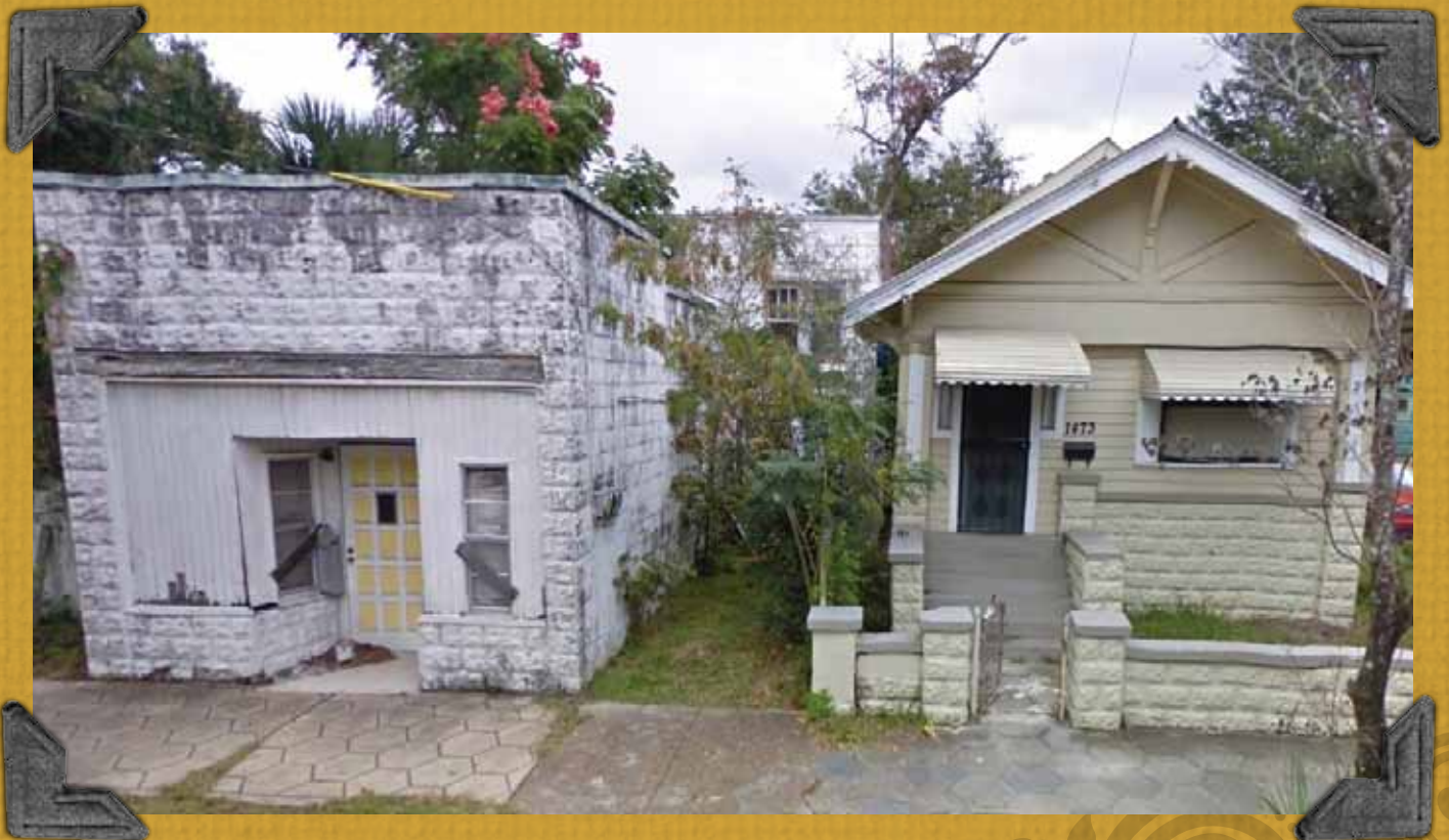
~ 1477 and 1473 Evergreen Avenue; The building on the left is the flower shop owned and operated by Blanche Hurston (demolished). The building on the right is the home originally owned by the Hurston family. ~
